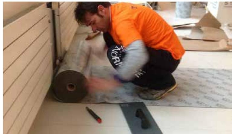
**DUAL FITTING SYSTEM** is an innovative dry system for laying large floor slabs (minimum recommended format 60x60 cm, thickness 1 cm). The DUAL FITTING SYSTEM provides adhesion between the slab and the support surface using a special blanket covered by a special adhesive applied on both sides.
