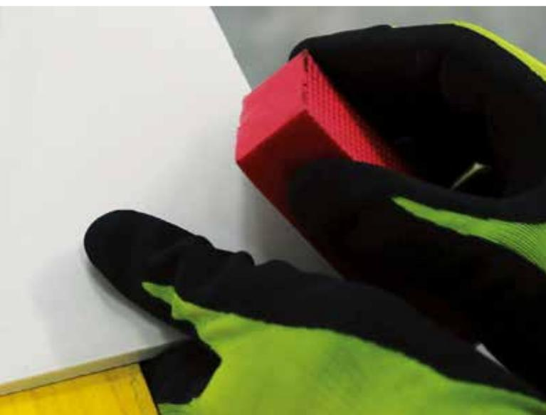
**THE FINISHING** of the edges on the cut side, if left visible, must be carried out using the special diamond buffer, or alternatively using appropriate resinous diamond discs.
